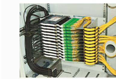
High-density subrack for Datwyler ODF, 3U
