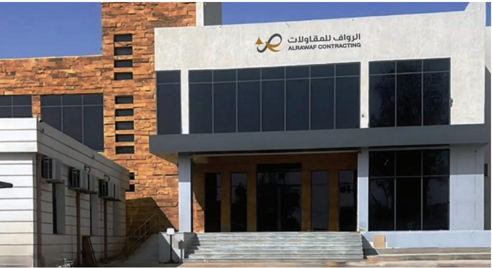
Al-Rawaf Contracting总部大楼
