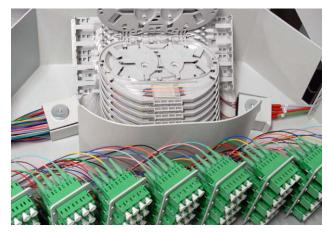
set up the cable ducts and insert the many different distribution and backbone cables. The PoPs have secured energy supplies. A ventilation and air conditioning system was also installed to dissipate the heat of the active components. ESR tasked a specialist company with the assembly and splicing of the fibre optic cables.
