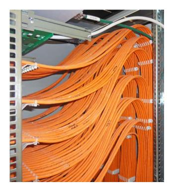
speed data transmission, but also incorporates the IP telephones, audio systems, video beamers and WLAN. The WLAN access points take the power they need via the data cables (PoE, Power over Ethernet).
