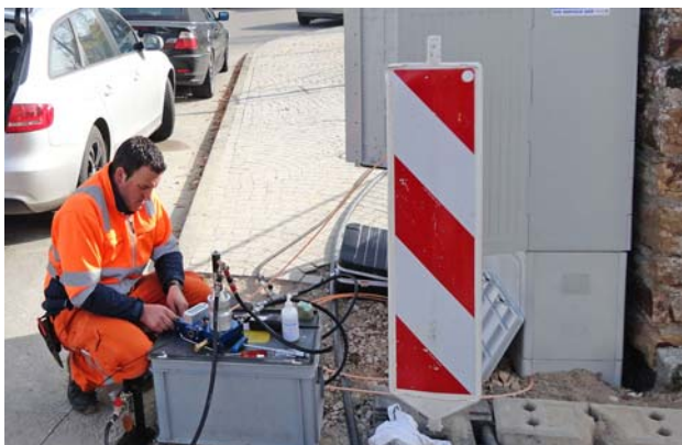
Image 1: Blowing fibre optic cables into ducts.
