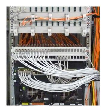
and single clips as well as innumerable special pins – offering system circuit integrity E30 and E90. Naturally, all the components have the necessary test certificates. These confirm that entire cable installation can be relied upon to continue to supply the connected safety systems with power for up to 30 / 90 minutes in the event of a fire.
