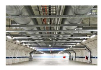
The zero halogen, low-smoke and flame-retardant safety cables are an integral part of the fire protection and safety concept. Amplit Oy installed these cables in the most important sub-buildings, the so-called upper storage and waste disposal yards, which are connected to the underground premises in the hospital area by way of several tunnels and shafts.
