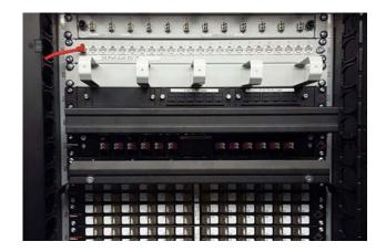
Datwyler's new 45 degree-angled type "KS-TA" RJ45 modules were used in the racks. In the fibre optic patch panels all the outgoing lines are also angled to left and right, allowing neat space-saving cable management at the front.
