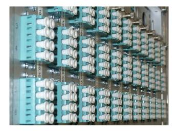
up with 1500 FO modules in 270 sub-racks with 4RU (including patch management tray) and in the server racks in 210 FO panels with 1RU. For the termination of the copper cables Datwyler supplied 135 3RU sub-racks with 1160 modular 6-port front panels and 285 1RU panels with 24 ports, depending on the rack type. There are also 13,300 FO duplex patch cables and 9100 copper patch cables for the connection of active devices.
