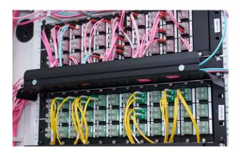
unaffected. All we have to do is replace the LC cassettes plug-and-play with MTP front panels. This means that we can save ourselves laborious splicing work," explained Anton Schultheiß of the local QSC Engineering and Network team.
