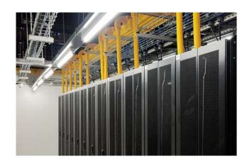
The use of different colours means that the subsystem and installed links are easily distinguishable.
